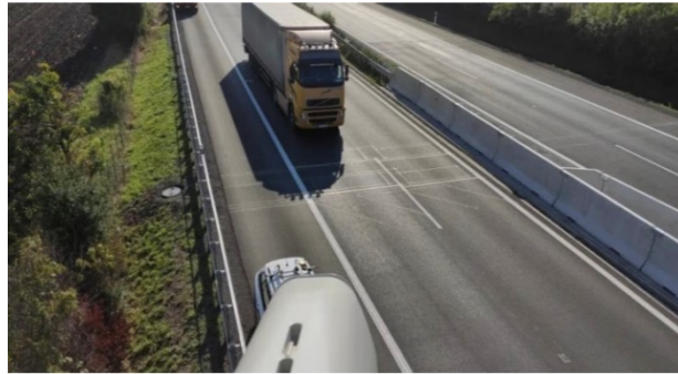
CrossWIM installed on a highway in Czech Republic
