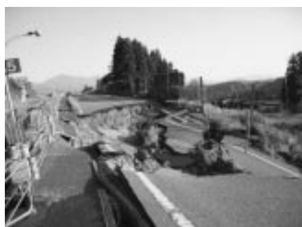
Chuetsu Earthquake (Collapsed lane on Kan-etsu Expressway) (Photograph: Japan Highway Public Corporation Hokuriku Branch)
